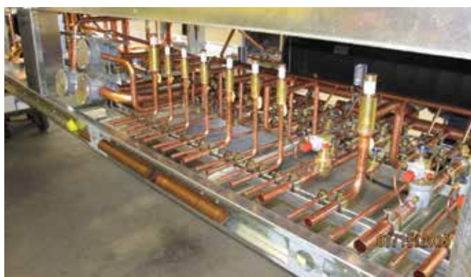
REFRIGERATION CIRCUITS UNDER LINK+ CONDENSER
