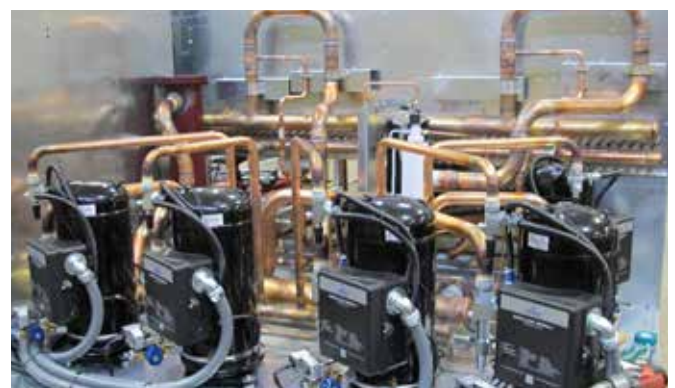
PARALLEL PIPED SCROLL COMPRESSORS
